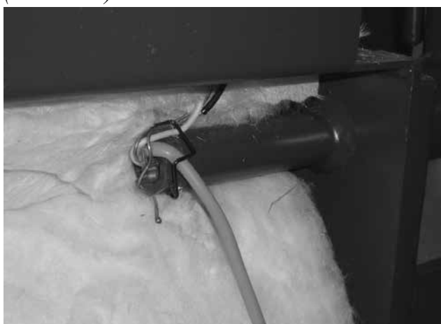
Fig. 15 – View of the water temperature sensor TK in the boiler pocket - DCxxSP(EP), or boilers with burner in the upper door - DCxxS(X), CxxS, ACxxS, DCxxRS
