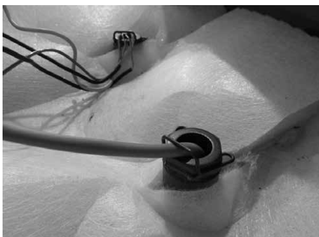
Fig. 16 – View of the water temperature sensor TK in the boiler pocket, DxxP, Pxx types
