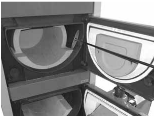
Open middle space of the boiler with a roof and example of ash removal with a poker
