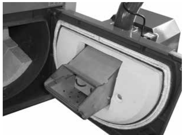
Open bottom door of the boiler during cleaning of the combustion chamber of the burner ATMOS A25
