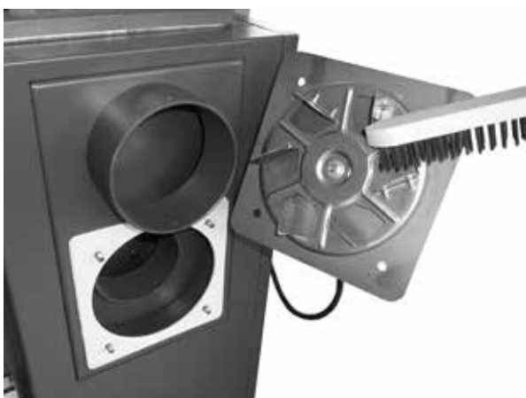
Sample cleaning of impeller and checking uprightness of vane on extract ventilator
